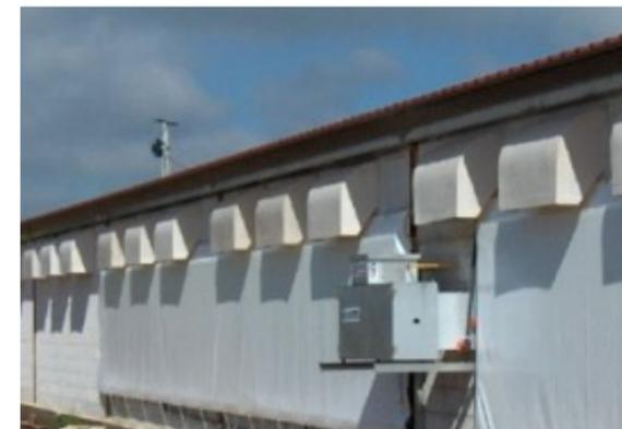
**ENG** The design allows the regulation at the entry, the speed and the direction of the air flow according to your needs. The inlet provides an optimum circulation of the air without streams. The aerodynamic of the flap makes better the air flow and prevents the falling when it comes inside the building.
