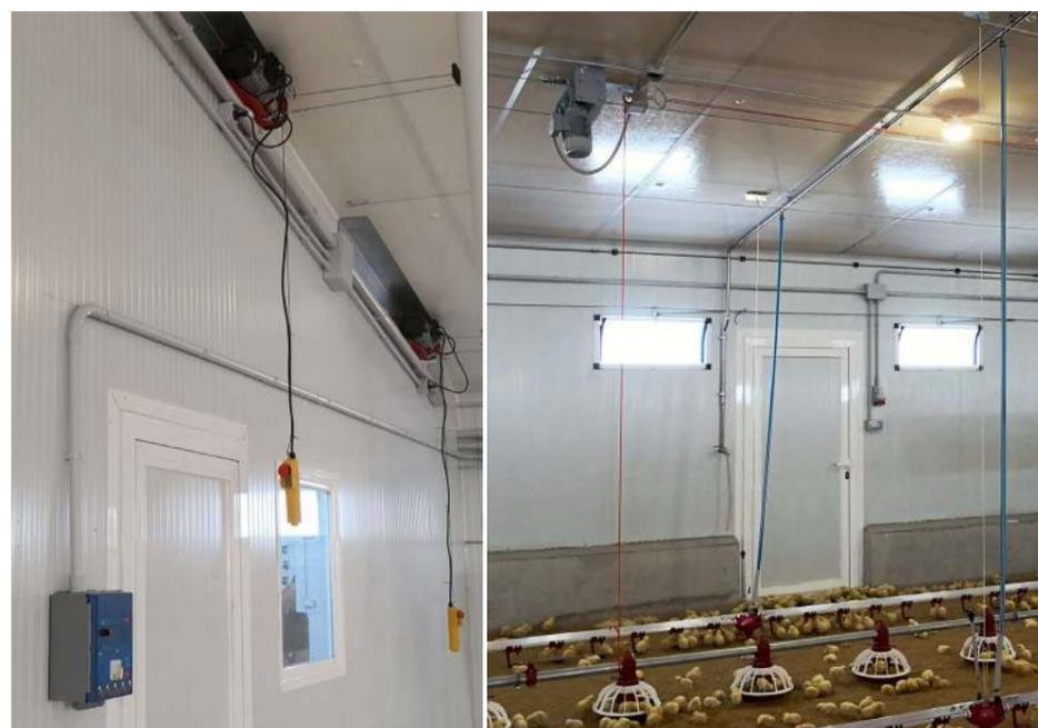
For better handling we propose an automatic lifting system with several built-in safety systems. The easiest way to adjust the feed level to the age of the birds with the push of a button. In addition to the automated option for line elevation, we offer electronic feed weighing management.
